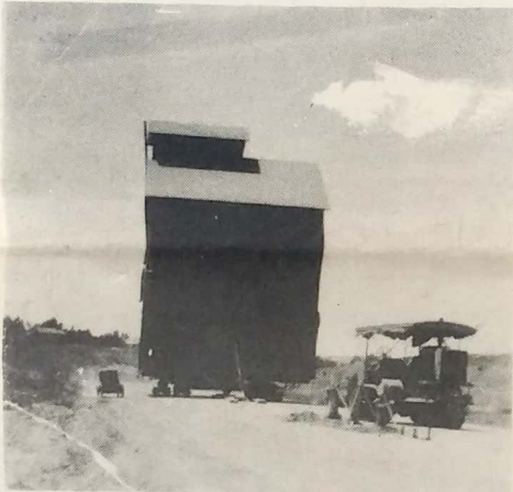
A GRAIN ELEVATOR gets moved to its new location, out of the way of the water soon to cover its former site.
