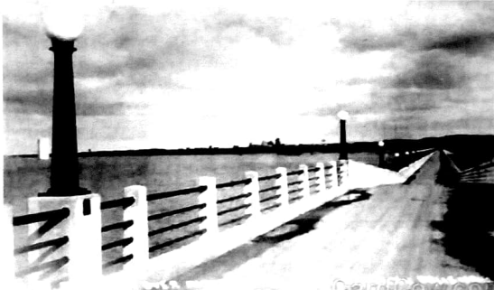
The bridge over the original American Falls Dam
