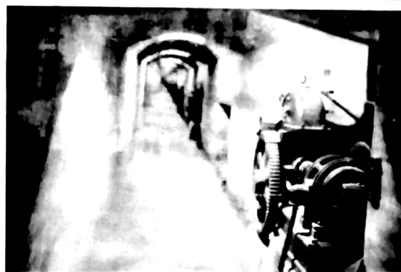
Inside the old dam
