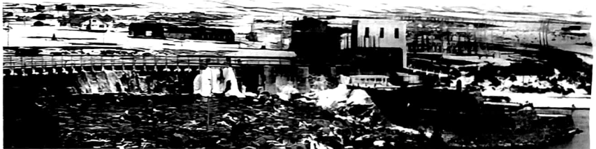
The powerhouse on the dam
