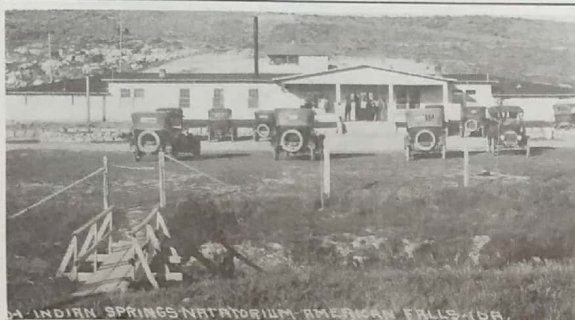
Above: Early look at Indian Springs Natatorium which is still in operation.
