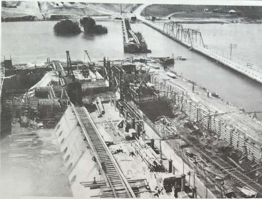
The dam under construction (above and above right)
