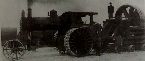
Steam powered harvesting in Power County
