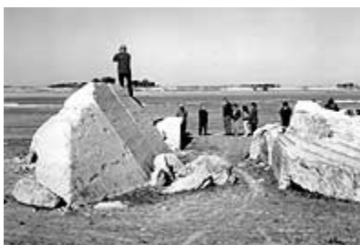
Culvert under the Oregon Short Line Railroad, Old American Falls townsite, (October, 1987).
